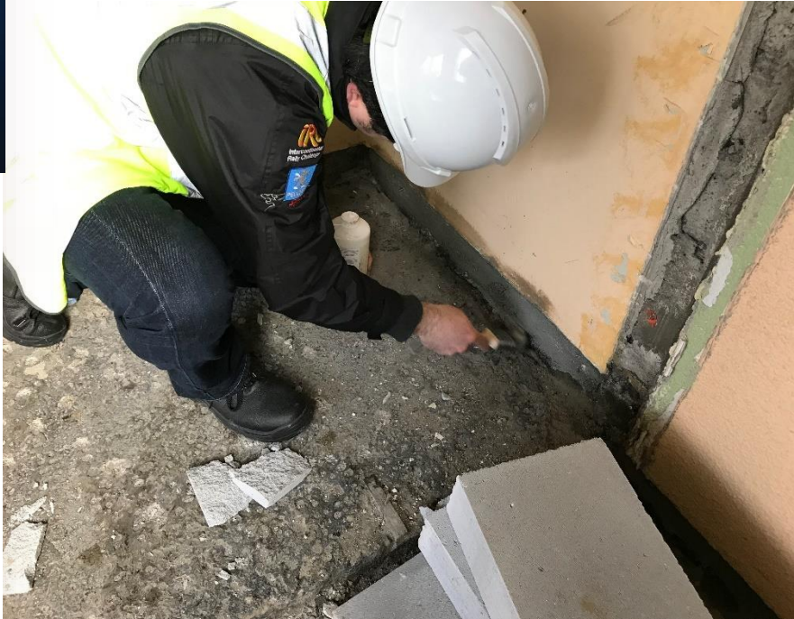
Floor to wall junctions, where surfaces are rough and preparation is essential
