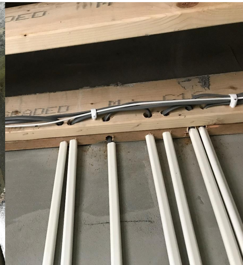
Multiple services passing through wood without specialist airtight grommets
