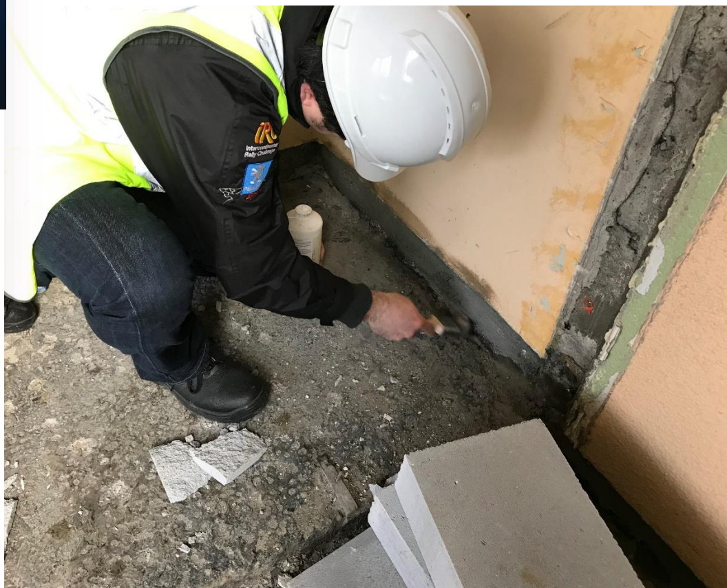
Remove dust and debris and apply primer prior to affixing tape
