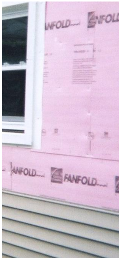
Insulation boards & tongue & groove cladding
