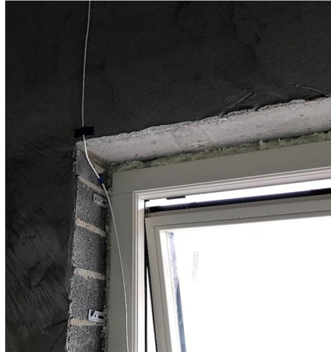
Window to wall connections
